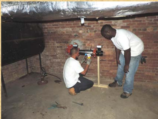
Outside and basement water line installation
